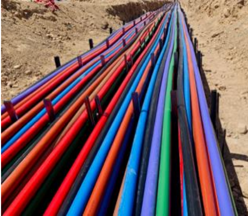
Data Center Trench Rack Design
